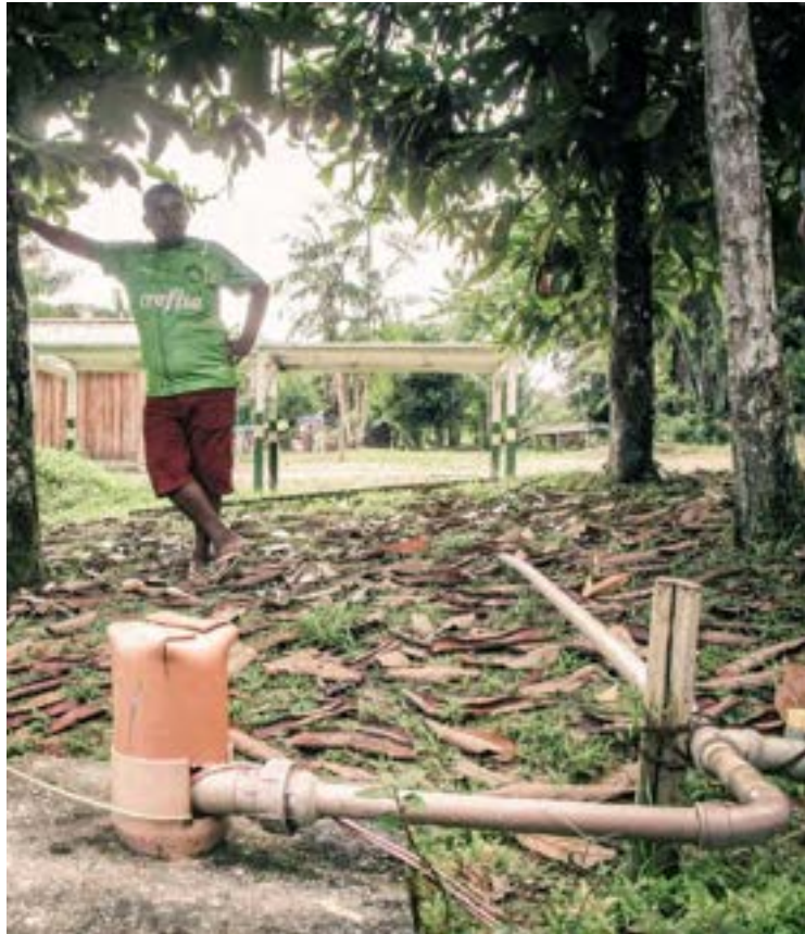
Solar-powered water pump for the village fountain in Cartúcho (MRN II)
